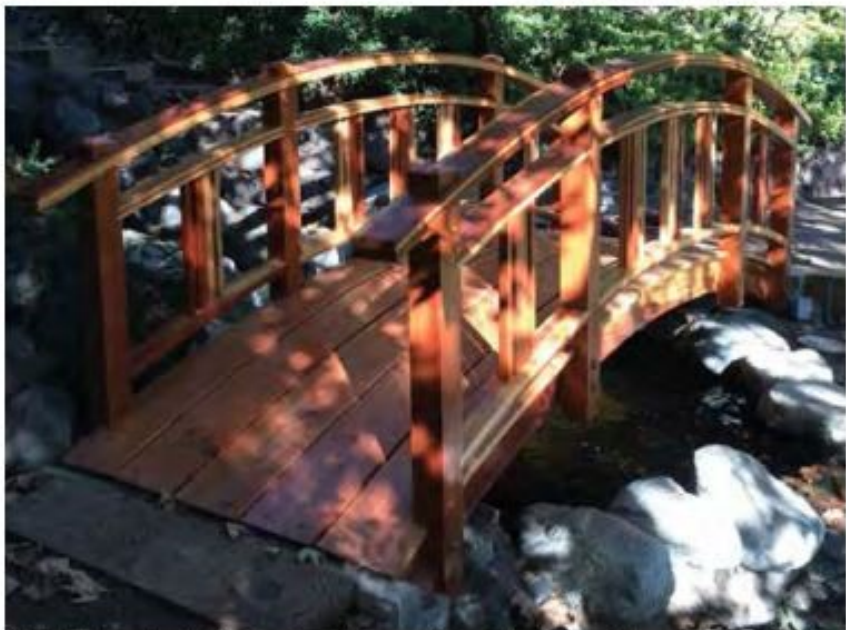
With help from friends, Macy laminated pieces of fir to make this graceful, arched footbridge. He now owns a very large number of clamps.
