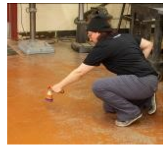
Testing the finished top
